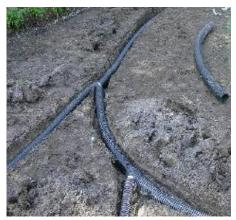
Buried drain extensions are used to catch water from your downspouts and move the water to an area away from your foundation.
