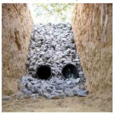
French Drains are used to catch water over a large surface area in the yard that is a low spot. The water is then moved to a desired area away from your foundation or towards a rain garden.
