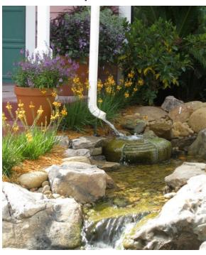
Dry river beds are used to catch water from your downspouts or low areas in the yard. Water is then transported to an area away from your foundation or into a rain garden. A dry river bed is the most attractive and ellegant way of moving water.
